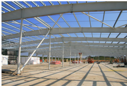
Frame under construction - Raciborz, Poland
