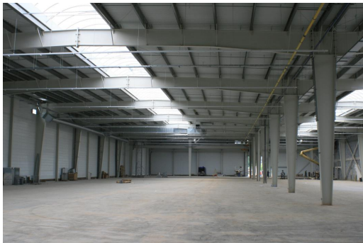
Frame under construction - Swidnica, Poland
